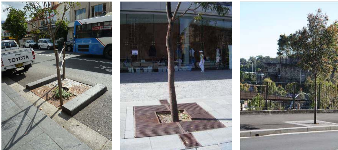
Figure 16: WSUD in Street Tree pits – Redfern St (left), Sydney University (centre) and Pirrama Park, City of Sydney (right) (Photos: Alluvium).
