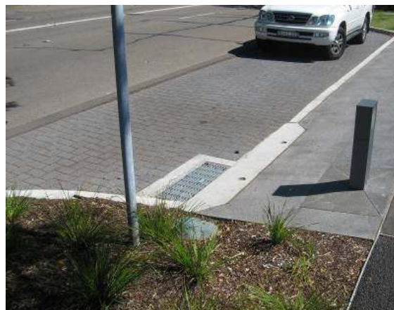
Figure 12: Porous concrete pavers at Rose Bay Promenade, Woollahra (Photos: Equatica)
