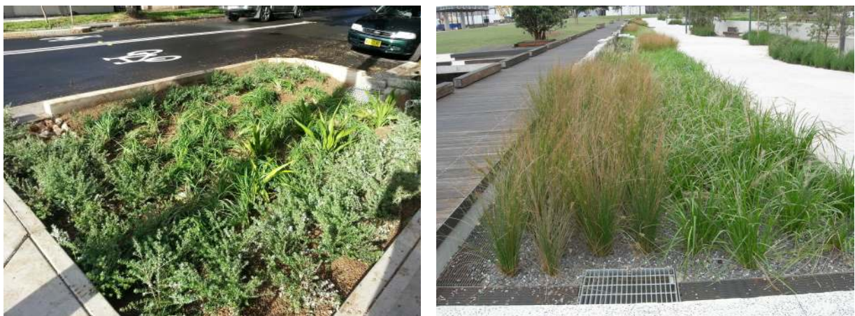
Figure 17: WSUD rain-gardens in The City of Sydney LGA – Telopea St, Redfern (left), Pirrama Park, Pyrmont (right), (Photos: Alluvium).
