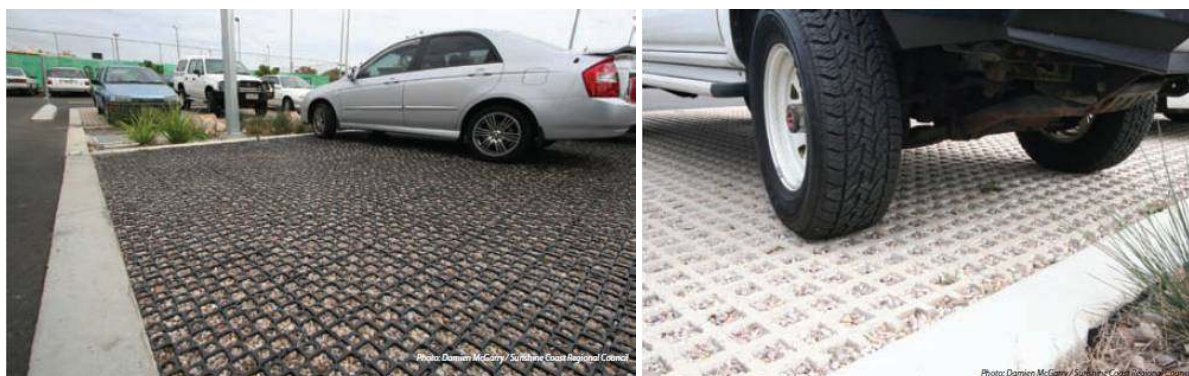
Figure 10: Gravel-filled lattices – heavy duty plastic (left) and concrete (right). (Photos: by Damien McGarry, Sunshine Coast Regional Council, as published in the Water by Design Concept Design Guidelines for Water Sensitive Urban Design ).
