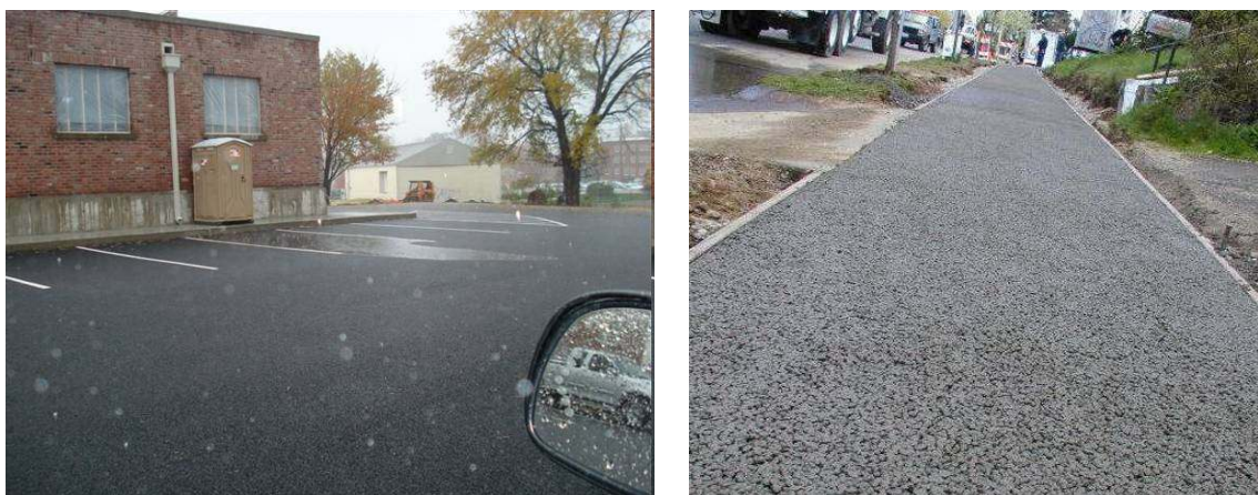
Figure 13: Porous asphalt (left) and porous concrete (right) pavements (Photos: http://www.christensen-construction.com/Porous Asphalt.html and http://www.perviouspavement.org/pervious_paths.htm )
