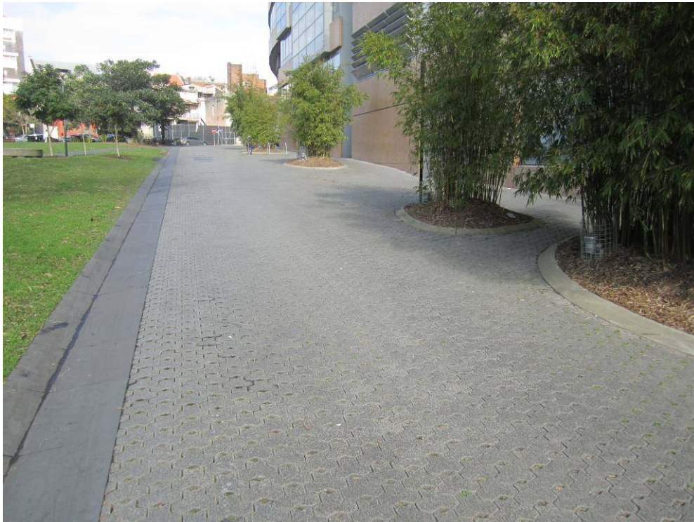
Figure 11: Open jointed porous pavers at Darlinghurst (Photo: Equatica)
