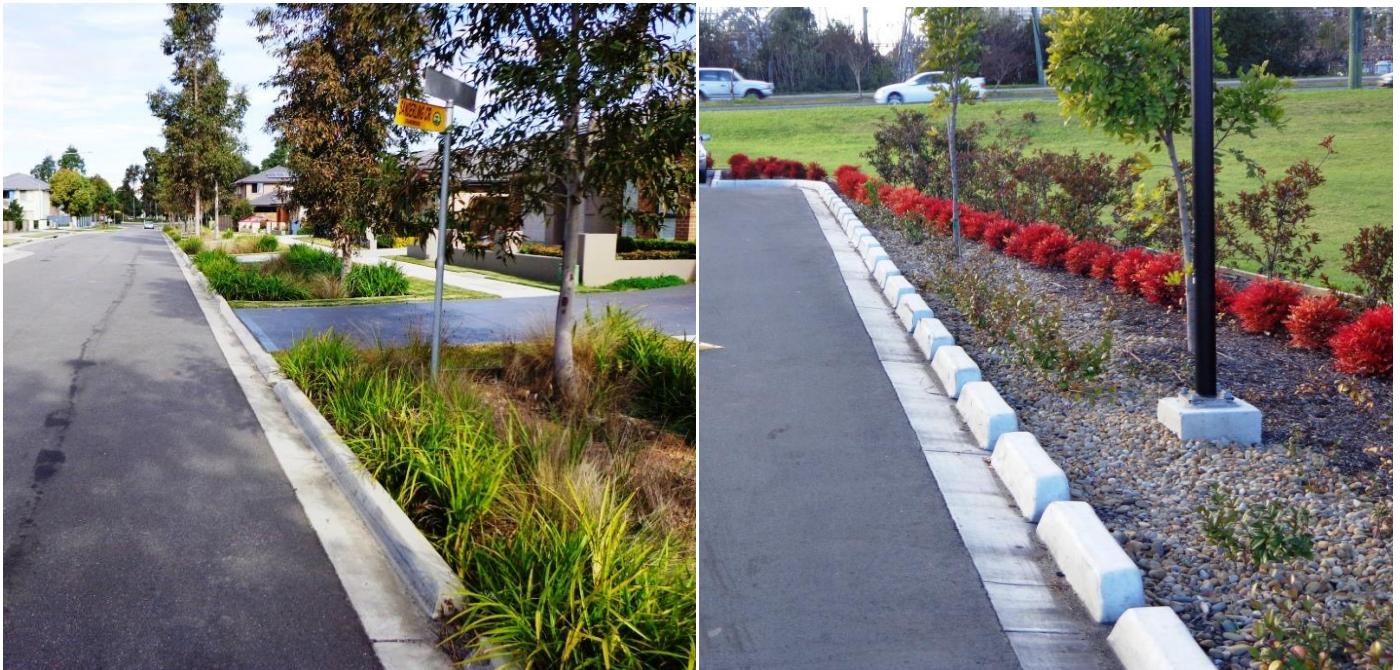
Figure 2: WSUD bioretention (Raingardens) basin in Carpark / Streets in Penrith LGA
