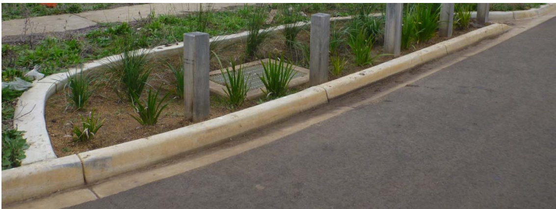
Figure 7 –Bioretention System/Raingarden in Estate on Aberline Road (Water Technology, 12/06/2013)
