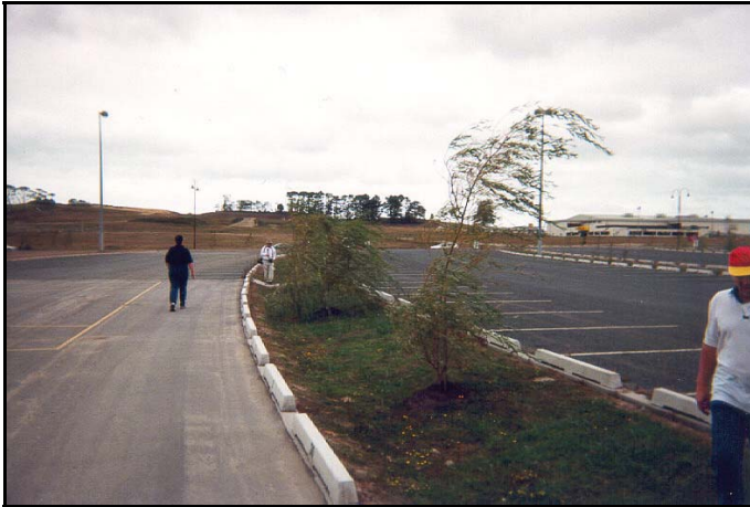
Figure 2 The use of vegetated medium strips for management of car-park stormwater runoff.
