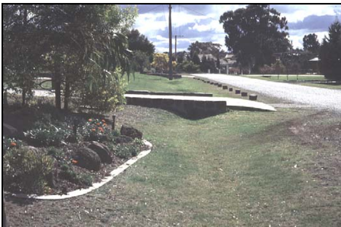
Figure 4 Grass swales in place of the conventional kerb and channel system for management of road runoff can promote both water quality improvement and flow attenuation.
