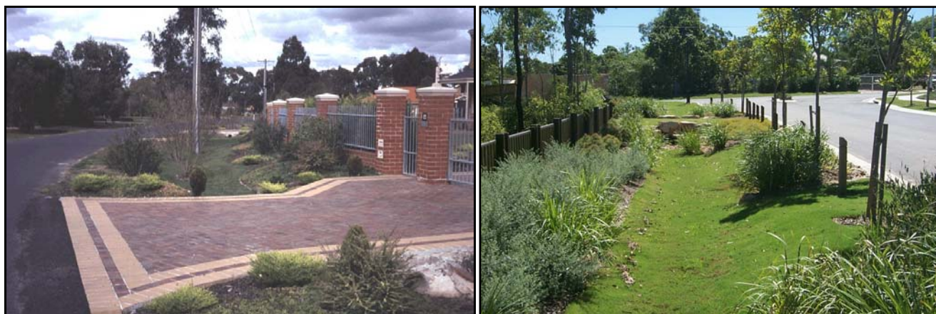
Figure 11 Grass swales are now increasingly being incorporated into residential streetscape as a landscape feature
