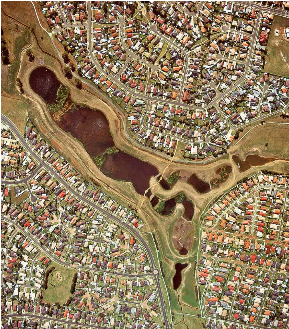
Figure 6 Constructed Stormwater Wetland built in 2000 at Hampton Park, Victoria, Australia (macrophyte zones will require at least two years to fully established)
