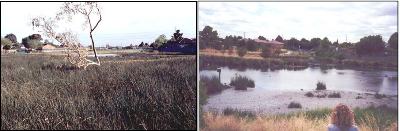
Figure 5 Constructed wetland in Melbourne without provision of a high flow by-pass and an inlet sedimentation zone : (Left) wetland fully established in 1997; (Right) wetland in 1999 – silted with sediment and a significant majority of vegetation scoured out by flood events.
