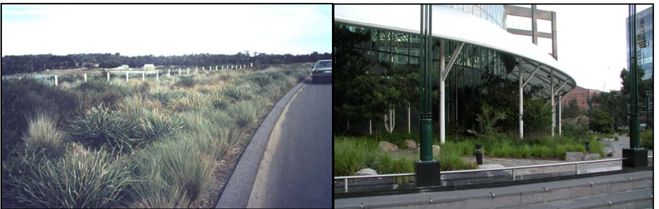
Figure 10 Constructed wetland systems can be used as source control measures along roads (left) and as part of an building forecourt (right).
