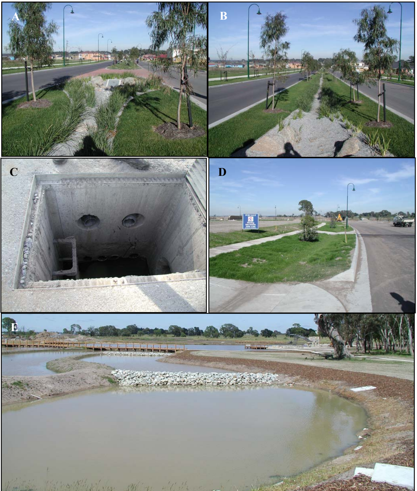
Figure 12 Features of the Lynbrook Estate stormwater management infrastructure (a & b) bio-filtration system constructed on the median strip of a divided road; (c) outlet pit of the biofiltration system showing the location of the perforated pipe beneath the biofiltration media; (d) a variation of the bio-filtration system is used for smaller undivided roads; (e) biofiltration system discharges into a constructed wetland for further stormwater quality improvement – ornamental lake in the background.
