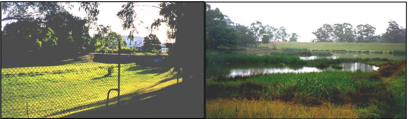
Figure 9 Conventional retarding basins (left) could be retrofitted (right) to provide a range of multiple functions without affecting its functionality as a flood mitigation facility
